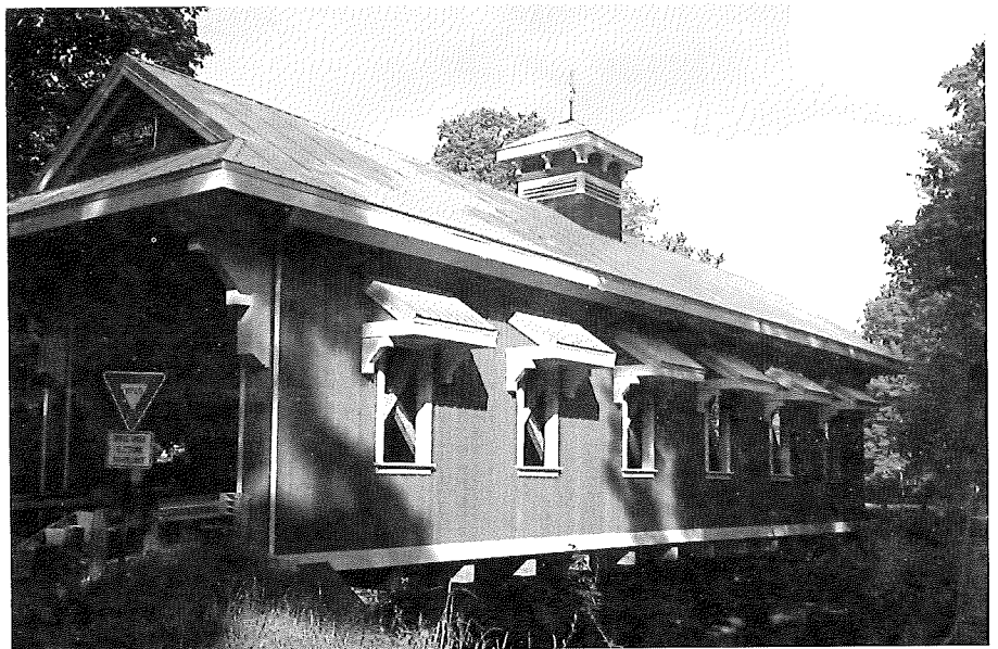
The John Eastman covered bridge, dedicated July 2014
